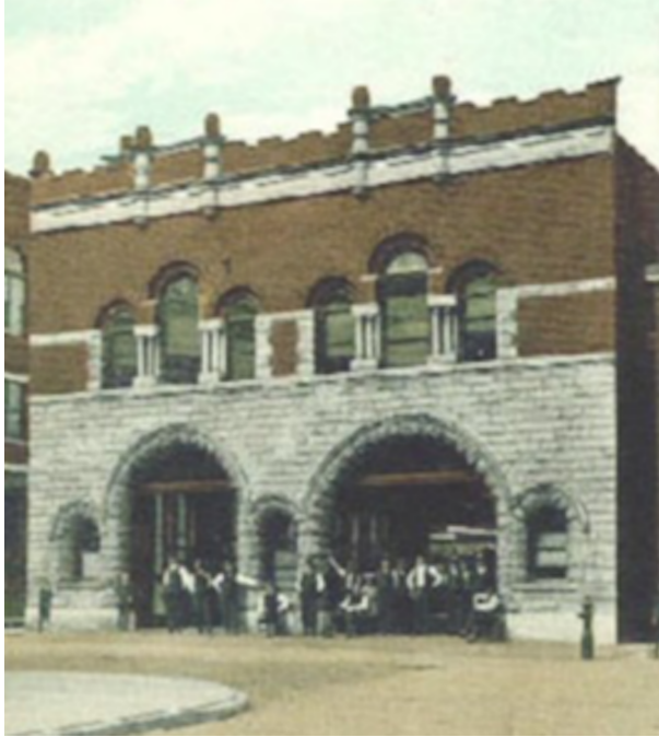
Company 1: Main Firehouse in Covington, KY until 1975
